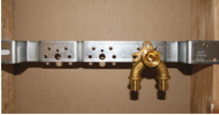
1 Fix bracket and mount fitting
