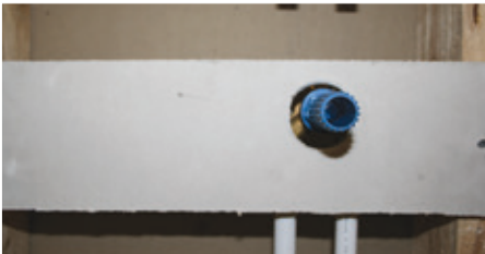
3 Finish the wall over the assembly
