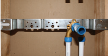
2 Connect pipe and pressure test
