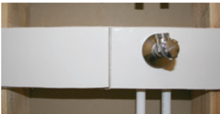
4 Connect tap to the BSP thread.
